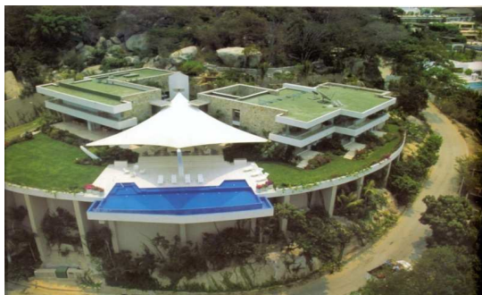
Plate 1: Aerial view of the Casa En Huatulco, Mexico, showing passive open spaces landscaping through its elevated suspended pool, green terraces at different levels and its green roof.
